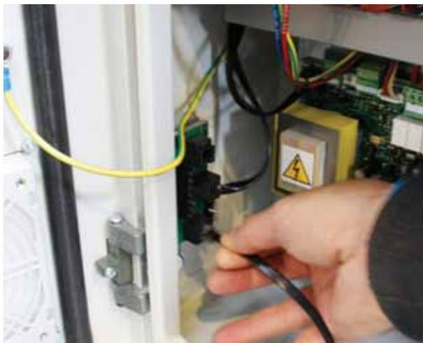
When several modules are installed, the p-lan network can be installed easily using quick connecting telephone wires (included in supply).
